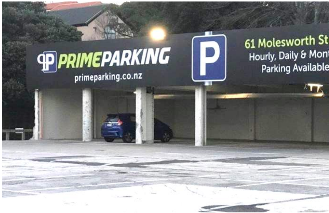
Photograph 2: Approximate location of former workshop and petrol tank in southwest corner of site. The petrol pumps were located immediately to the right of the middle column.
