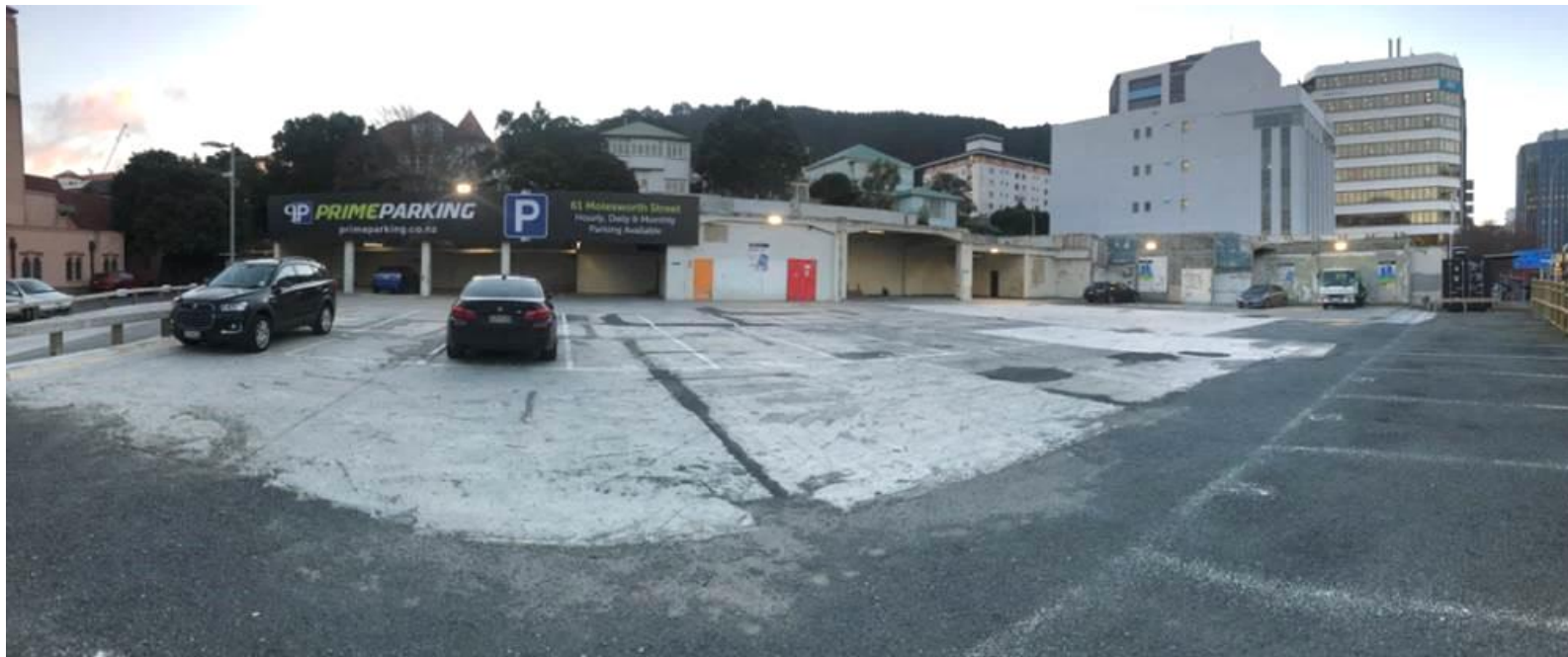
Photograph 1: Panorama of site showing former workshop area (PrimeParking sign above), substation (red door) and plantroom and fuel storage room (black door opening) at the rear of the site, with Molesworth Street visible to the far right. The rear wall and associated workshop and services areas are aligned approximately north-south.
